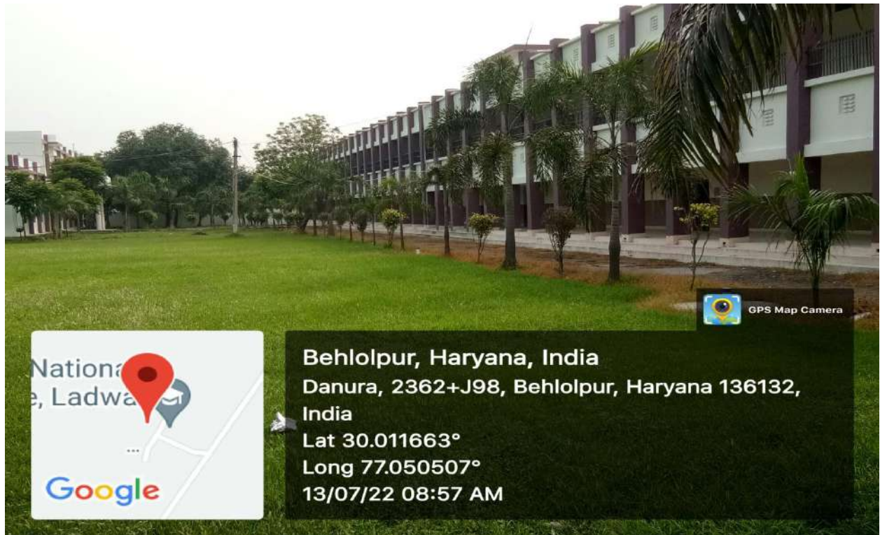
Figure 13: landscaping with trees and plants in the inside Lawn
