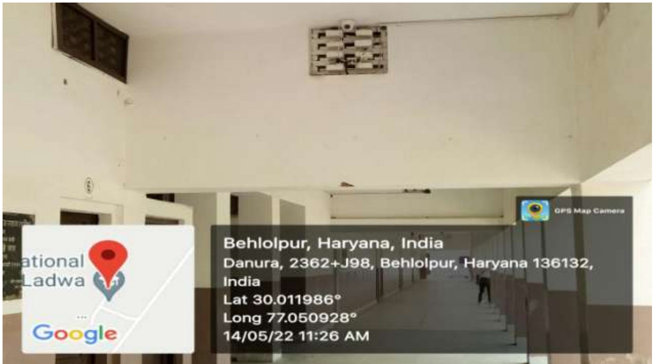
Figure 2: Surveillance Camera, Ground Floor Corridor
