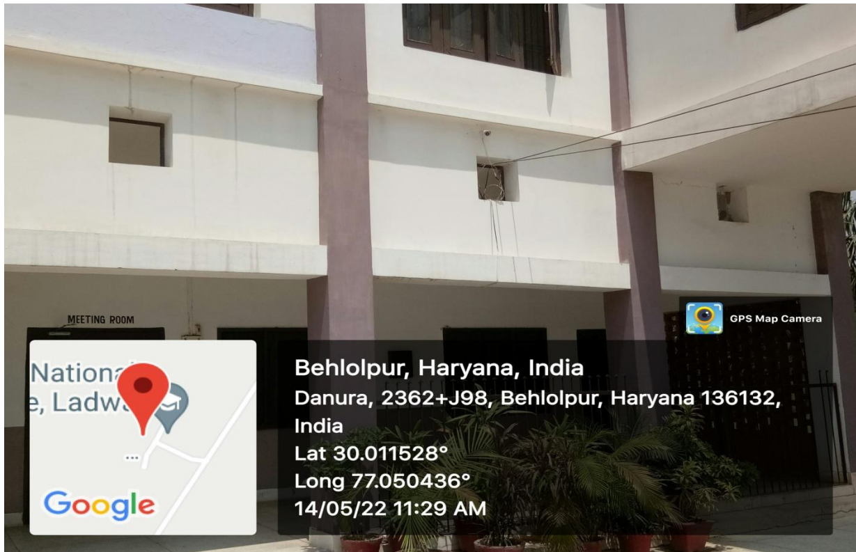
Figure 3, Surveillance Camera, Outside Open Area
