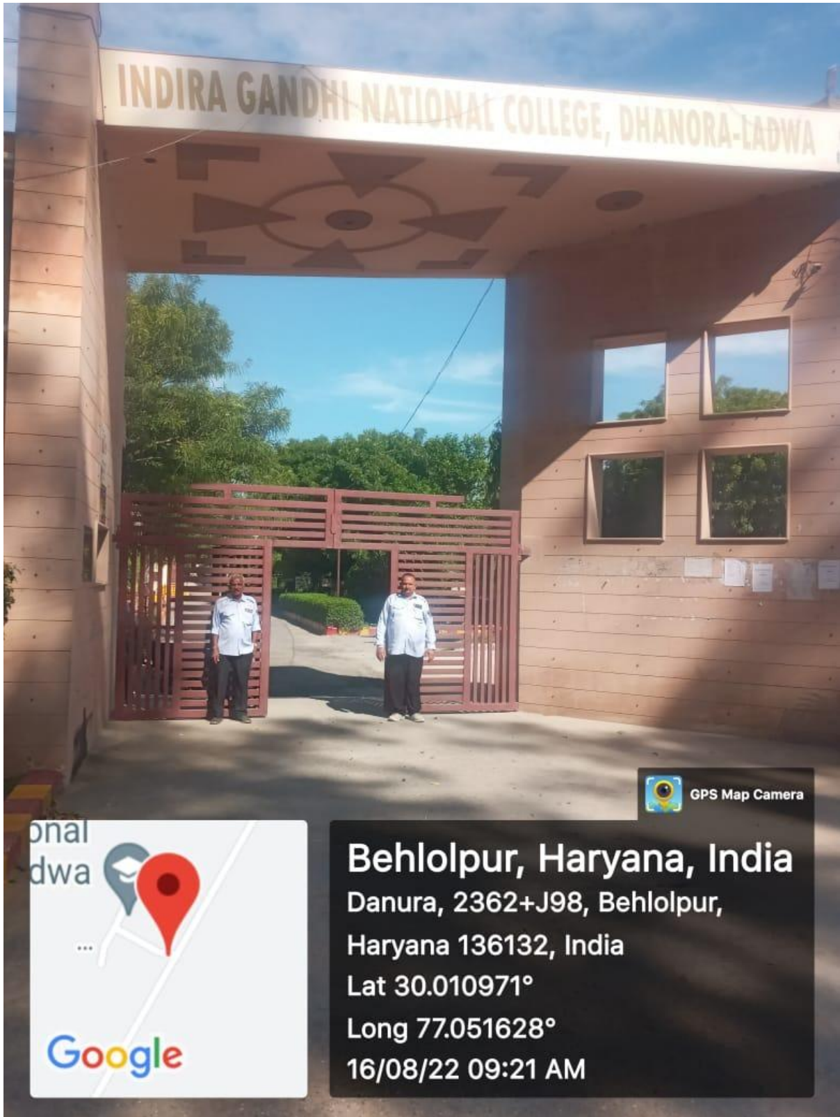
ii. High boundary Wall
