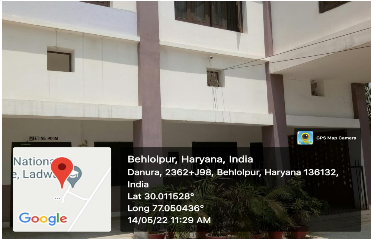
Figure 3, Surveillance Camera, Outside Open Area
