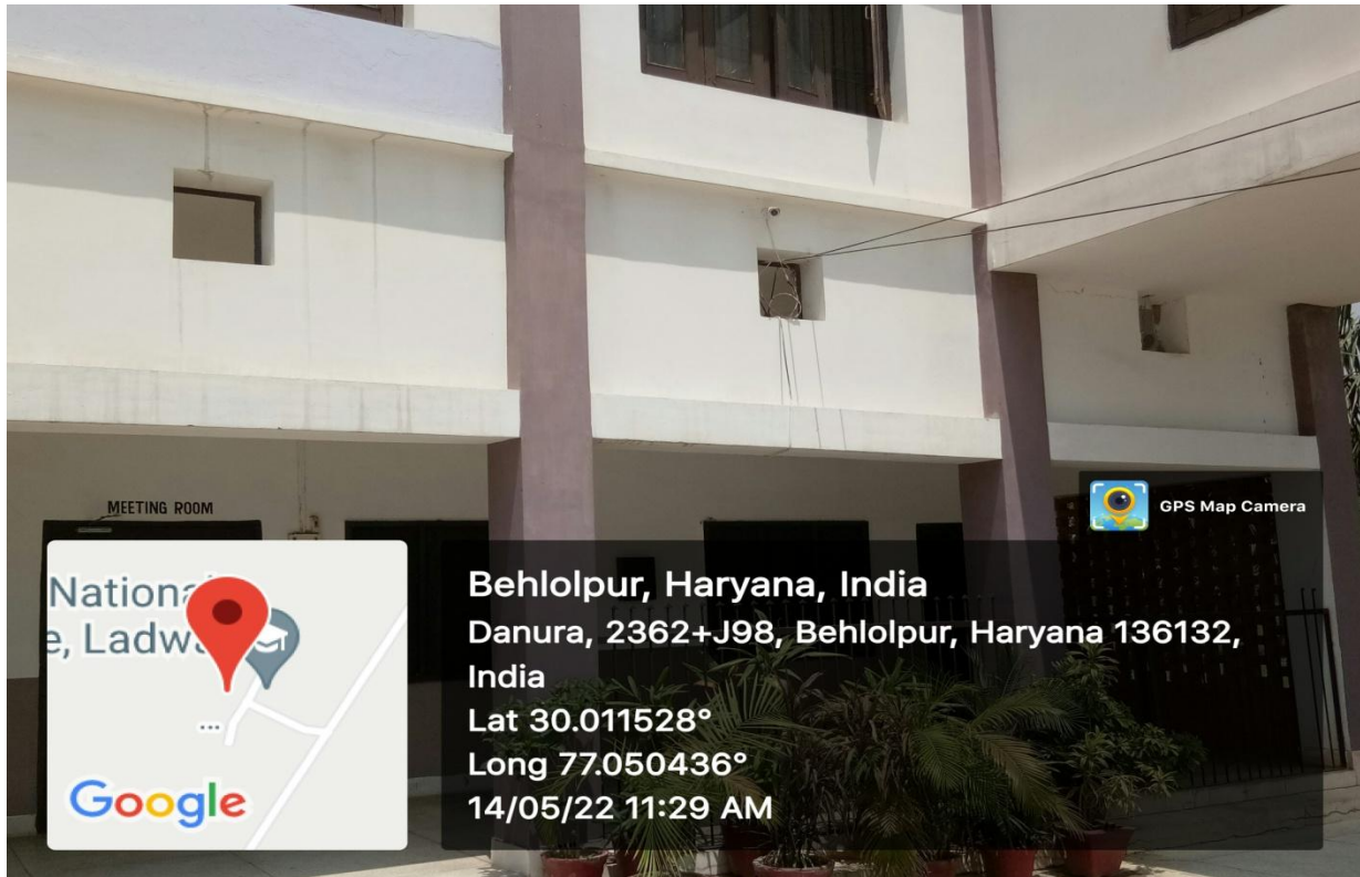
Figure 3, Surveillance Camera, Outside Open Area
