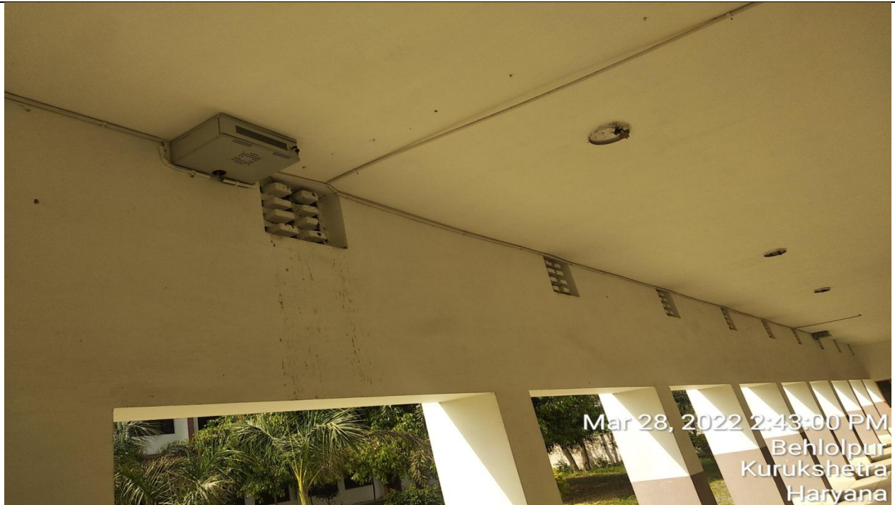
4.1.3 Smart Classroom with projector, screen, wi-fi etc.
